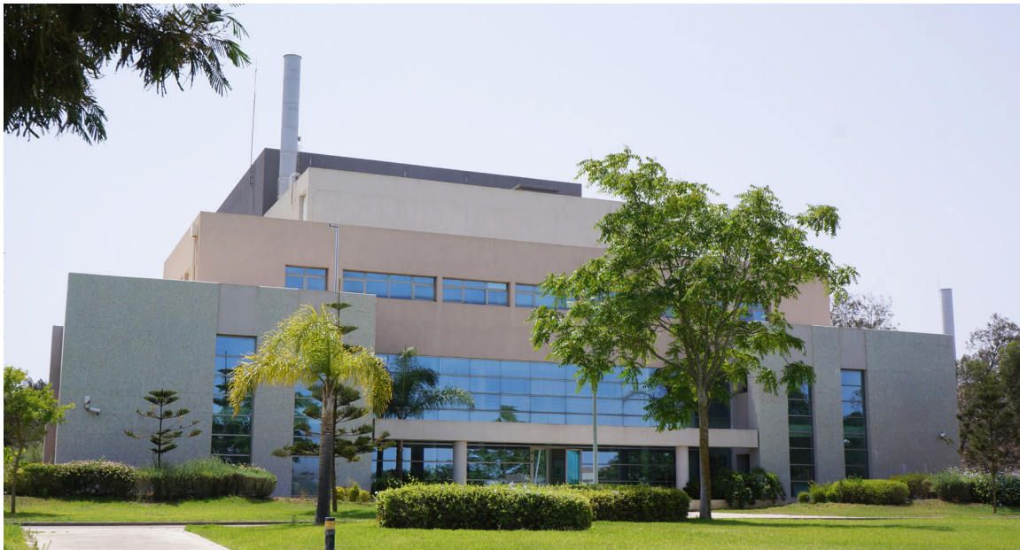
Nuclear Research Reactor Building
